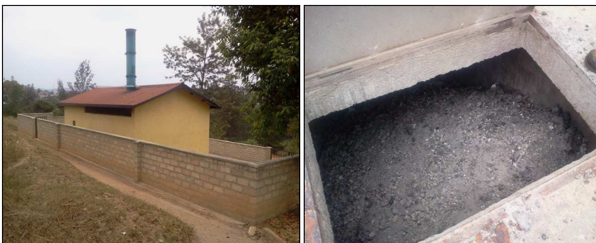
Figure 11: Incinerator at King Faisal Hospital (left picture) and Ash waste disposal in a concrete pit (right picture).
