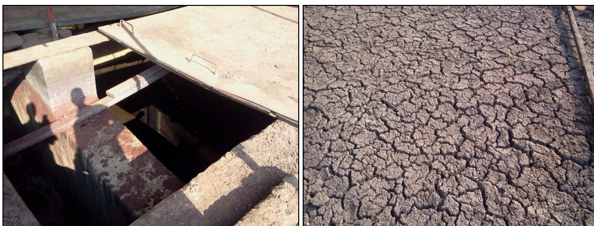
Figure 14: Two septic tanks of a capacity of 80\text{ m}^3 holding a toxic chemical wastewater from the paint process (left picture). Dried sludge from the septic tanks (right picture)
