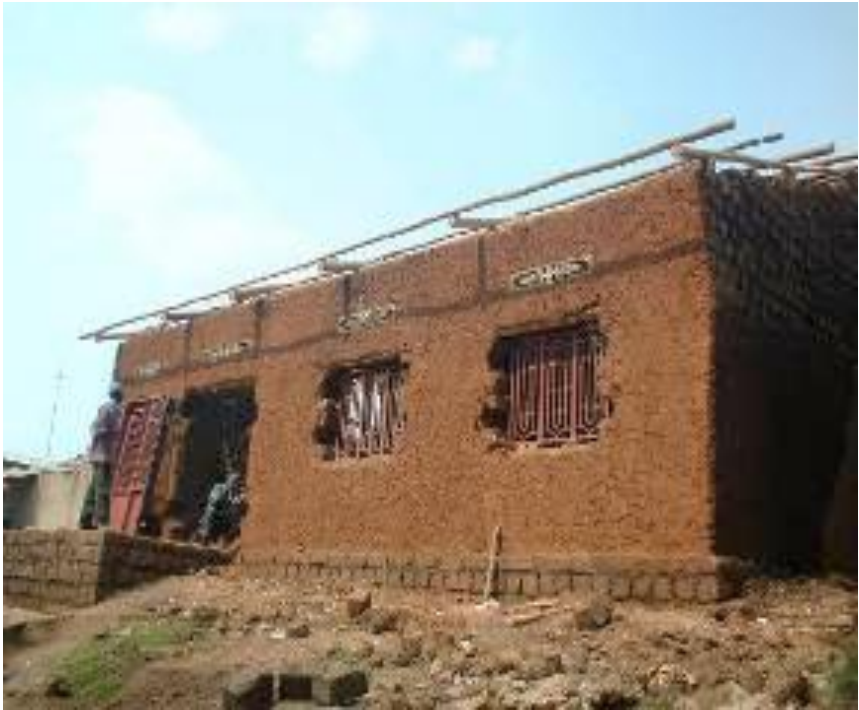
FIGURE 6-4 TRADITIONAL ADOBE HOUSE BEFORE PUTTING ROOFING
