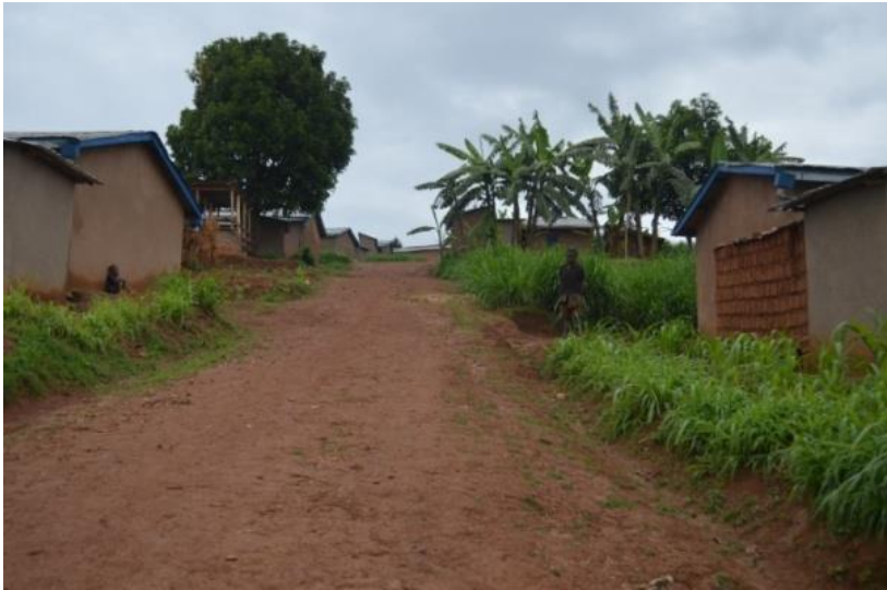
FIGURE 6-2 ACCESS ROAD ALONG THE SETTLEMENT
