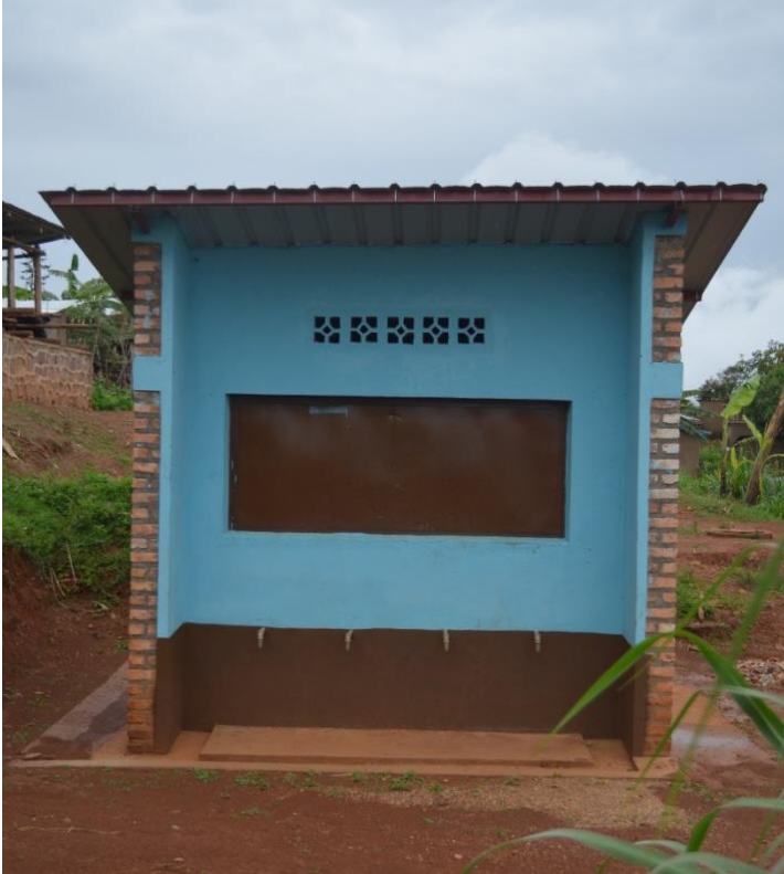
FIGURE 3-5 COMMUNITY DRINKING WATER TAP IN MUYEBE VILLAGE
