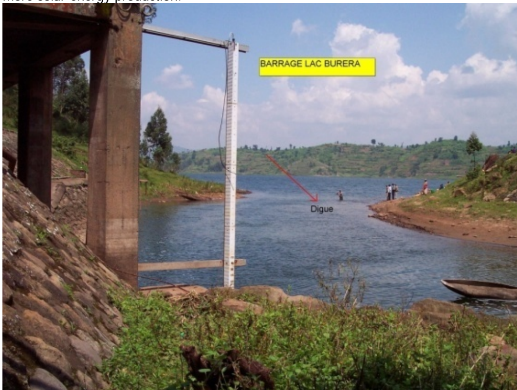
Figure 26 Water level decline on Lake Burera which supplies Hydroelectric plants of Ntaruka and Mukungwa
