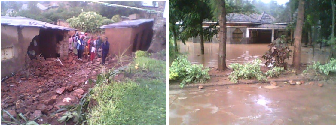
Figure 30 Destruction of unplanned urban (Kigali) settlement due to heavy rains and Floods in the Hotel La Palisse compound (Photo of 23 rd January 2010)
